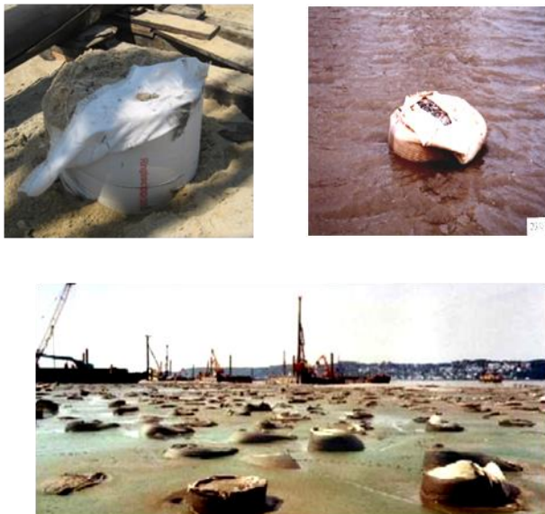
Figure 8. Examples of completed GECs: in a sand platform, in streaming water, in sludge.
