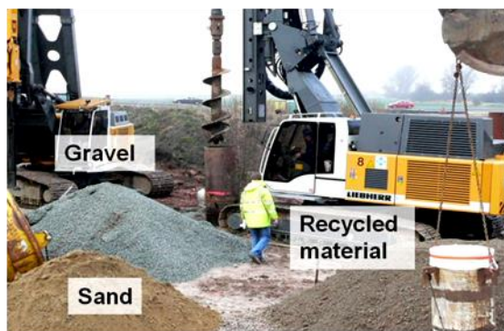
Figure 5 Different fills for GEC in a field trial.
