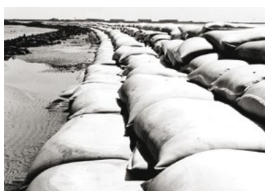
1963 Rüstersieler Watt Germany Dike construction SoilTain® Bags
