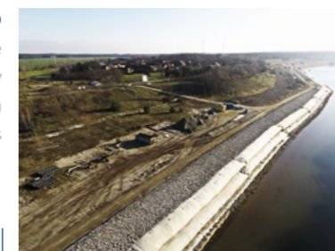
2016 Sedlitzer See Germany Cliff stabilisation SoilTain® Tubes
