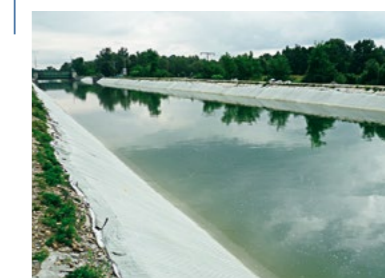
2013 Mittlere-Isar-Kanal Germany Canal refurbishment Incomat® Standard
