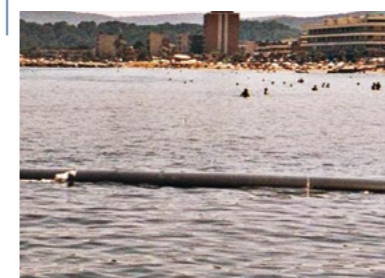
2002 Le Lavandou France Breakwaters SoilTain® Tubes
