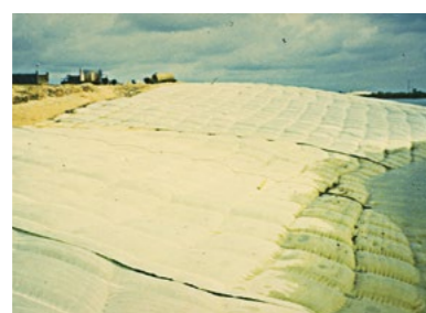
1983 Warri River Nigeria Revetment Incomat® Flex
