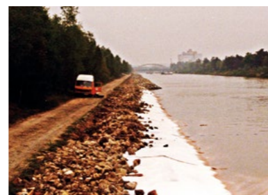
1989 Mittellandkanal Germany Revetment HaTe® Nonwovens
