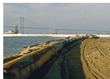
1986 Wilmington Harbour USA Land reclamation Stabilenka®
