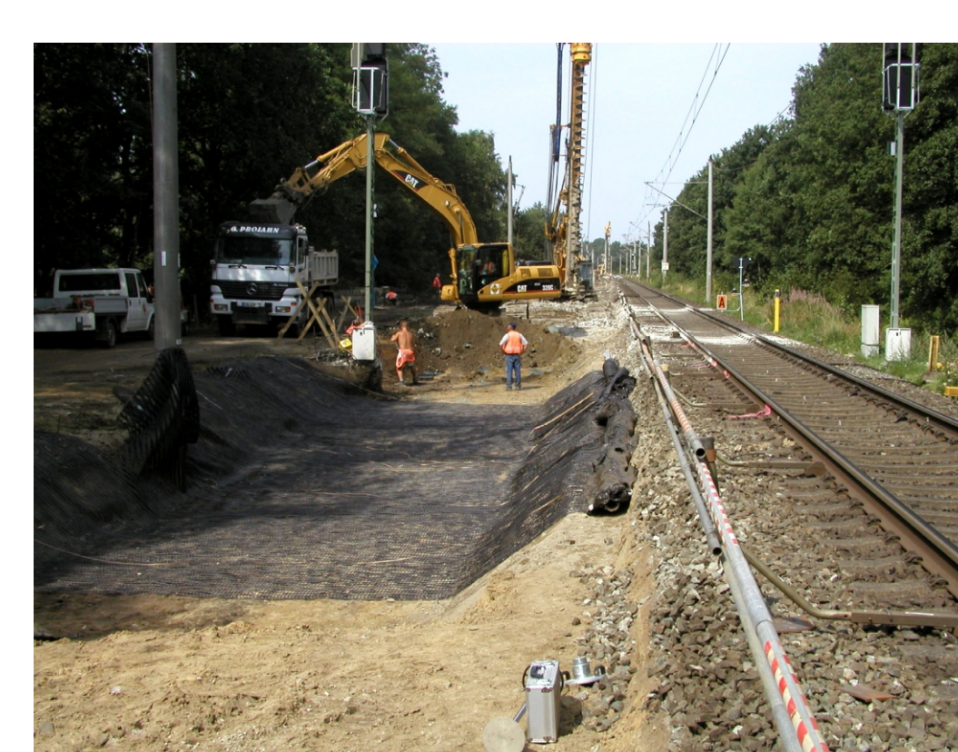
Railroad embankment on piles, Büchen, German Rail (DB), 2003
