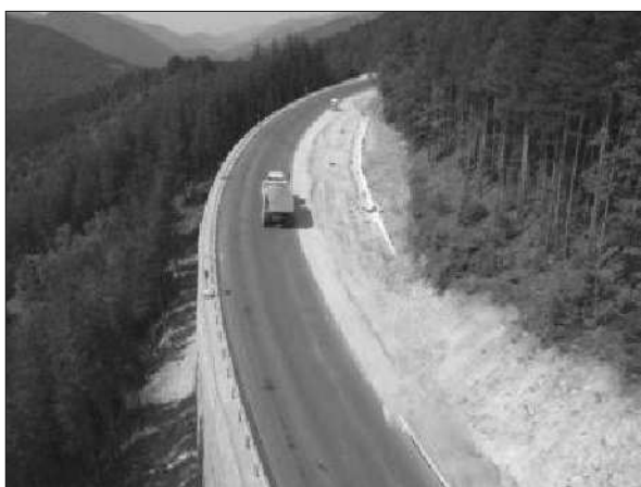
Figure 9. Top view of a completed GRS-wall.
