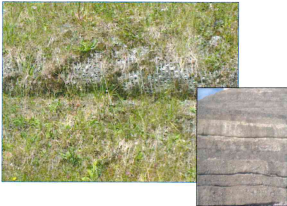
Fig. 11. August 2014: left: zoom of a vertical layer of the geogrid facing with a “belly”; right: same section in September 1994.
