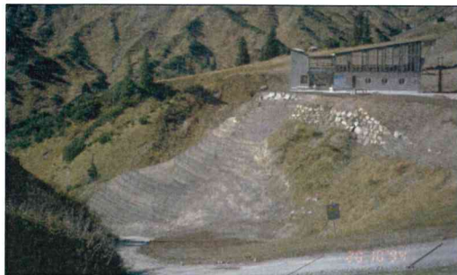
Fig. 7. Geogrid reinforced landslide stabilization just after completion (end of September 1994).
