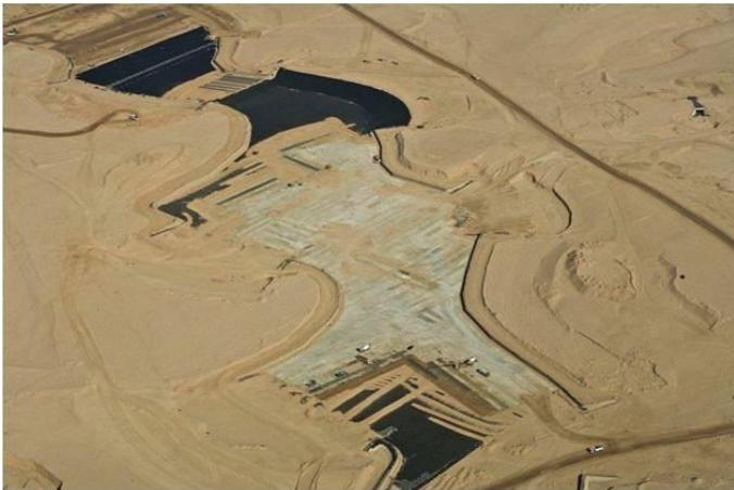
Figure 10. aerial photo – laid geotextile membrane partly with concrete covering
