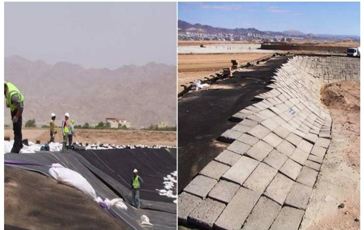
Figure 12. Sealing and covering the sealing sheet behind the reinforced earth block.
