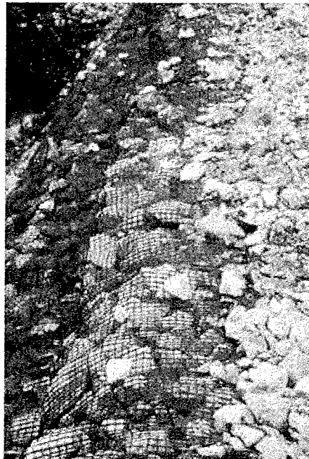
Figure 12 : “Federal Road B 227” – Extremely coarse fill confined by flexible geogrids
