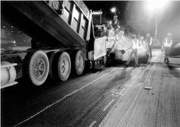
**FIGURE 7 Installation of the Polyester Reinforcement Grid In 2000**
