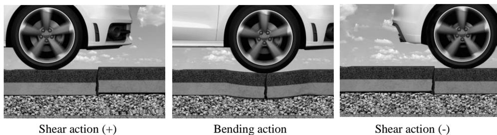
**FIGURE 1 Critical Loading Cases in a Pavement Crack**
