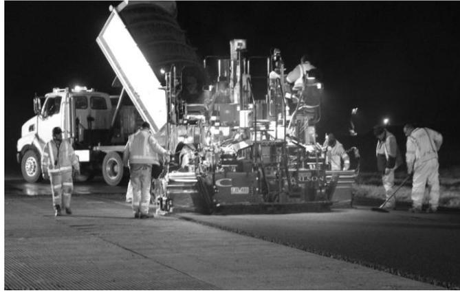
**FIGURE 11 Laying Asphalt Over the Polyester Asphalt Reinforcement**
