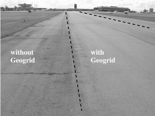
**FIGURE 5 Overview of the Studied Section: View of the Taxiway to the Maintenance Hangar**
