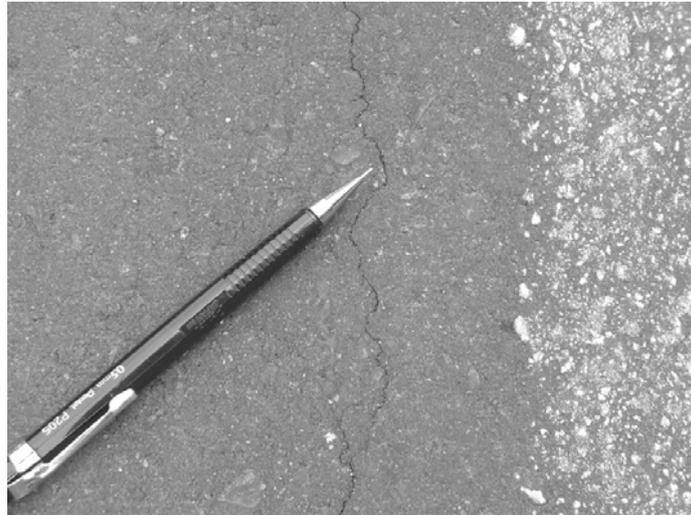
Figure 7: Early reflective cracking (March 2013)
