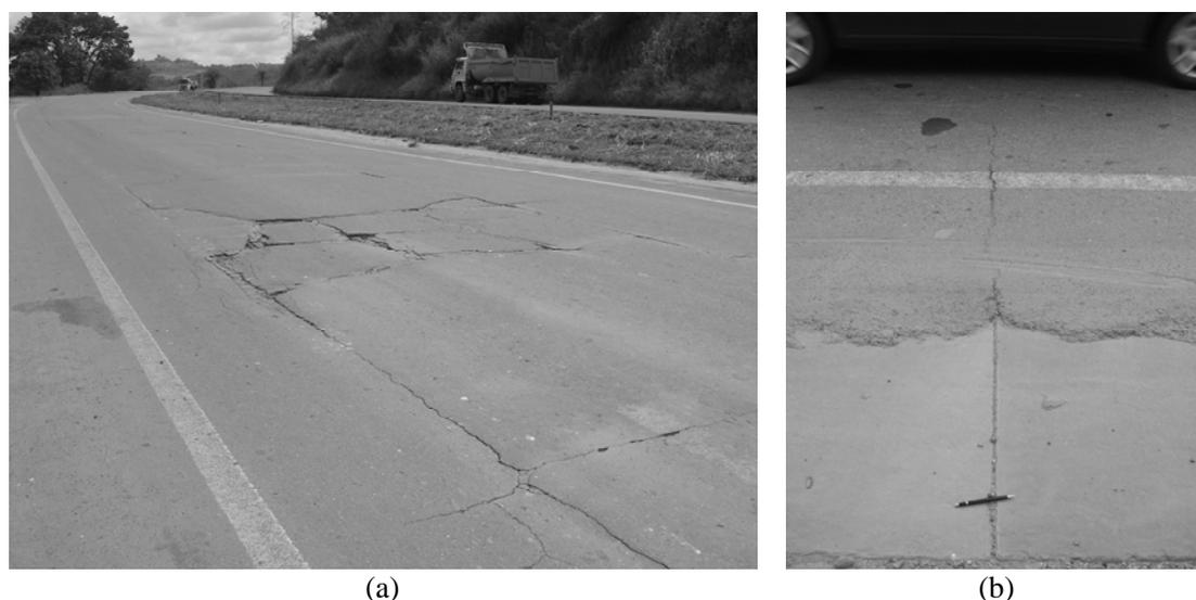
Figure 1: Joints and cracks of the concrete slabs propagated to the surface (December 2012)
