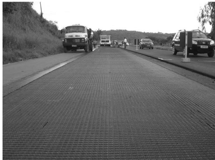
Figure 8: HaTelit® asphalt reinforcement
