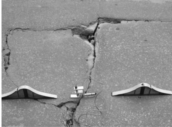
Figure 4: Crack and corner break at station 163
